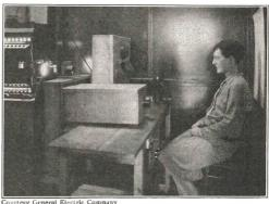
A CLOSE-UP OF THE TELEVISION TRANSMITTER, SHOWING THE ARRANGEMENT OF THE PHOTO-ELECTRIC CELLS
